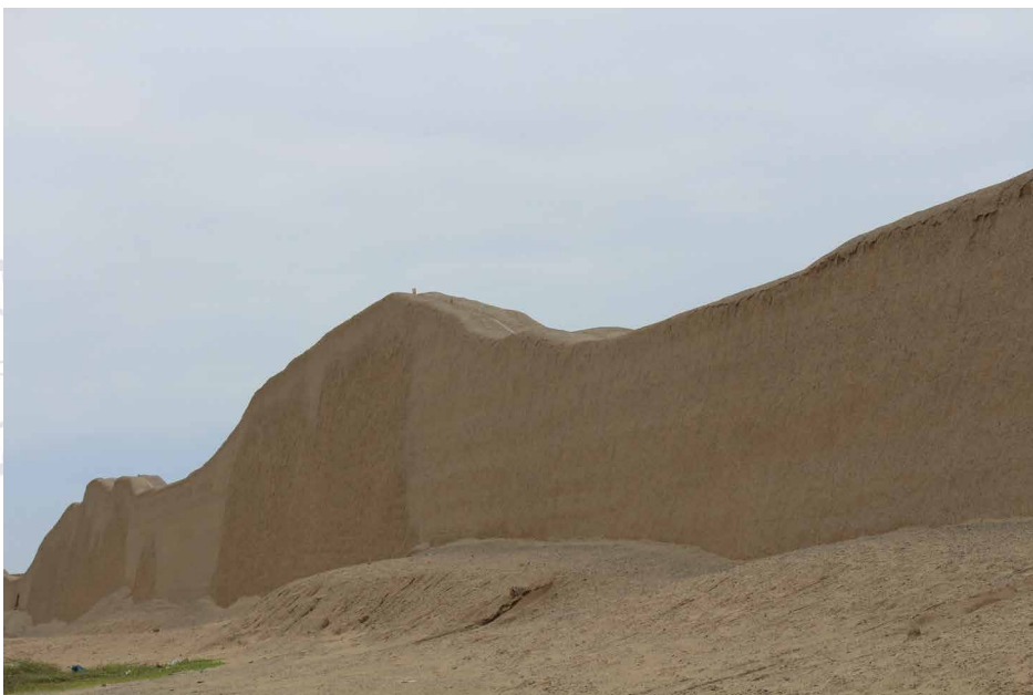
Exterior wall restored part of a walled enclosure Chan Chan
